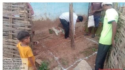
➤ **Foundation Excavation:** Foundation Excavation Completed for 30 out of 100 toilets.
